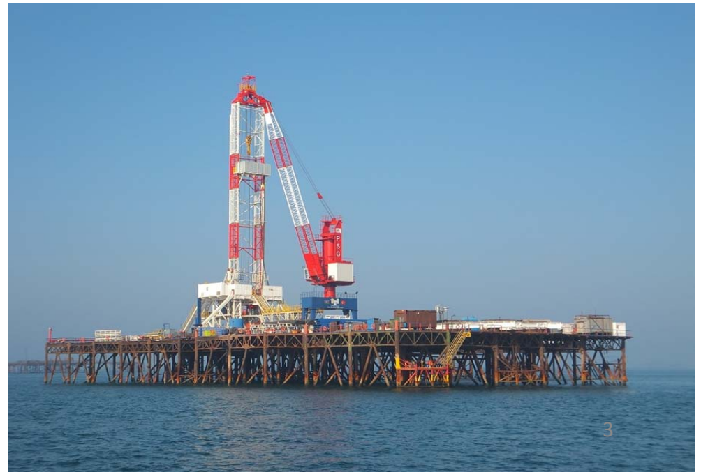
PSG 2 Rig on BH029 Platform
