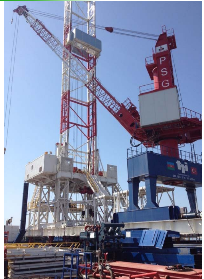
PSG 1 Rig on GD Platform 2
